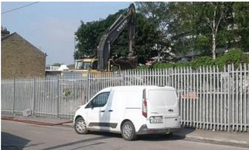
Demolition of Saint Andrews Court is now complete.
