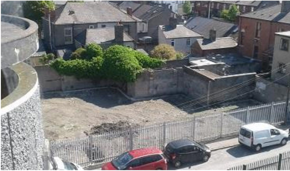
Collapsed drain issue within site at Sackville now resolved for all households affected.
