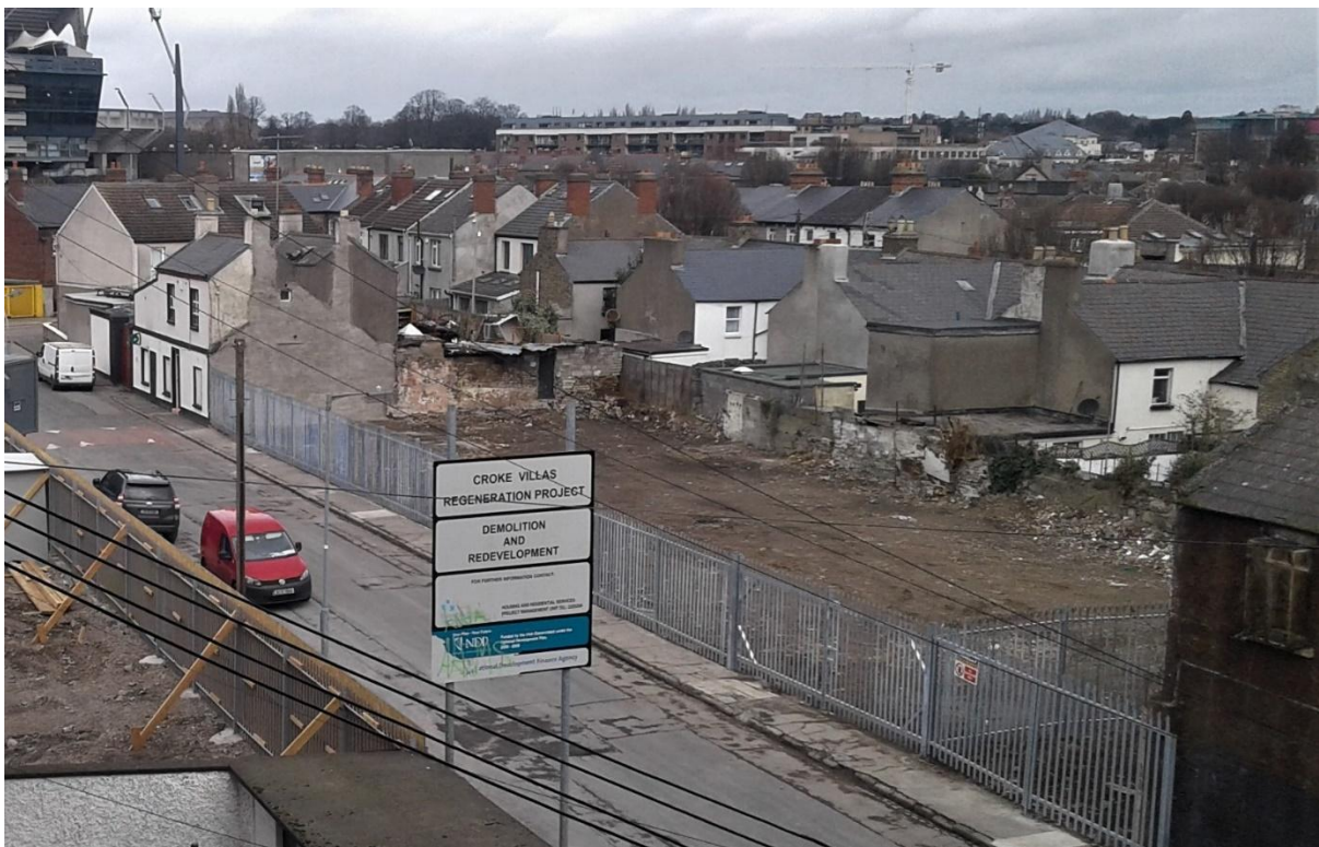
Demolition work on the former cottages on Sackville Avenue is now complete and the two sites cleared.
